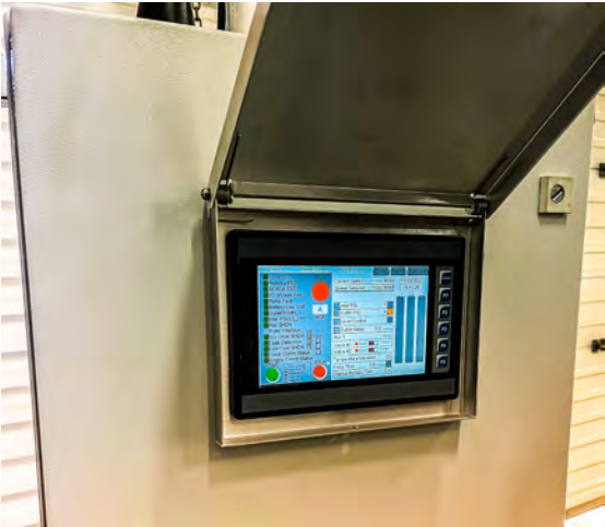
Trial at Petronas of new automated pipeline valve control - improving safety & reducing manpower
